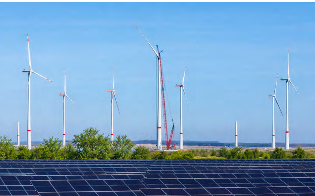
Renewable energy sites under construction: Forst-Briesnig II wind farm and Bohrau solar park
