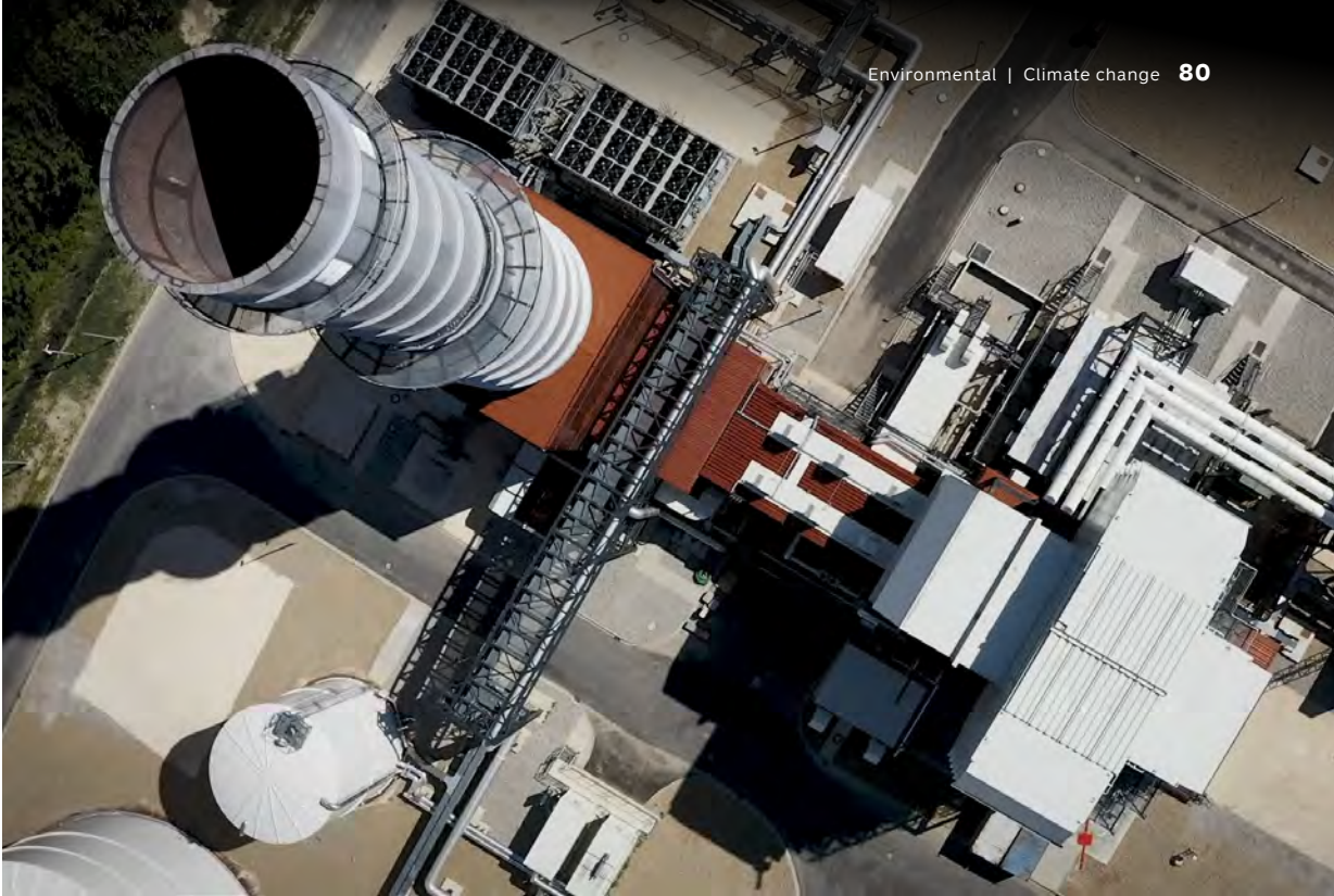
Leipheim gas-fired power plant in Bavaria
